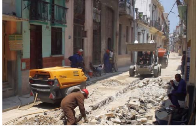
Digging up Tejadillo Street, third day of performance
